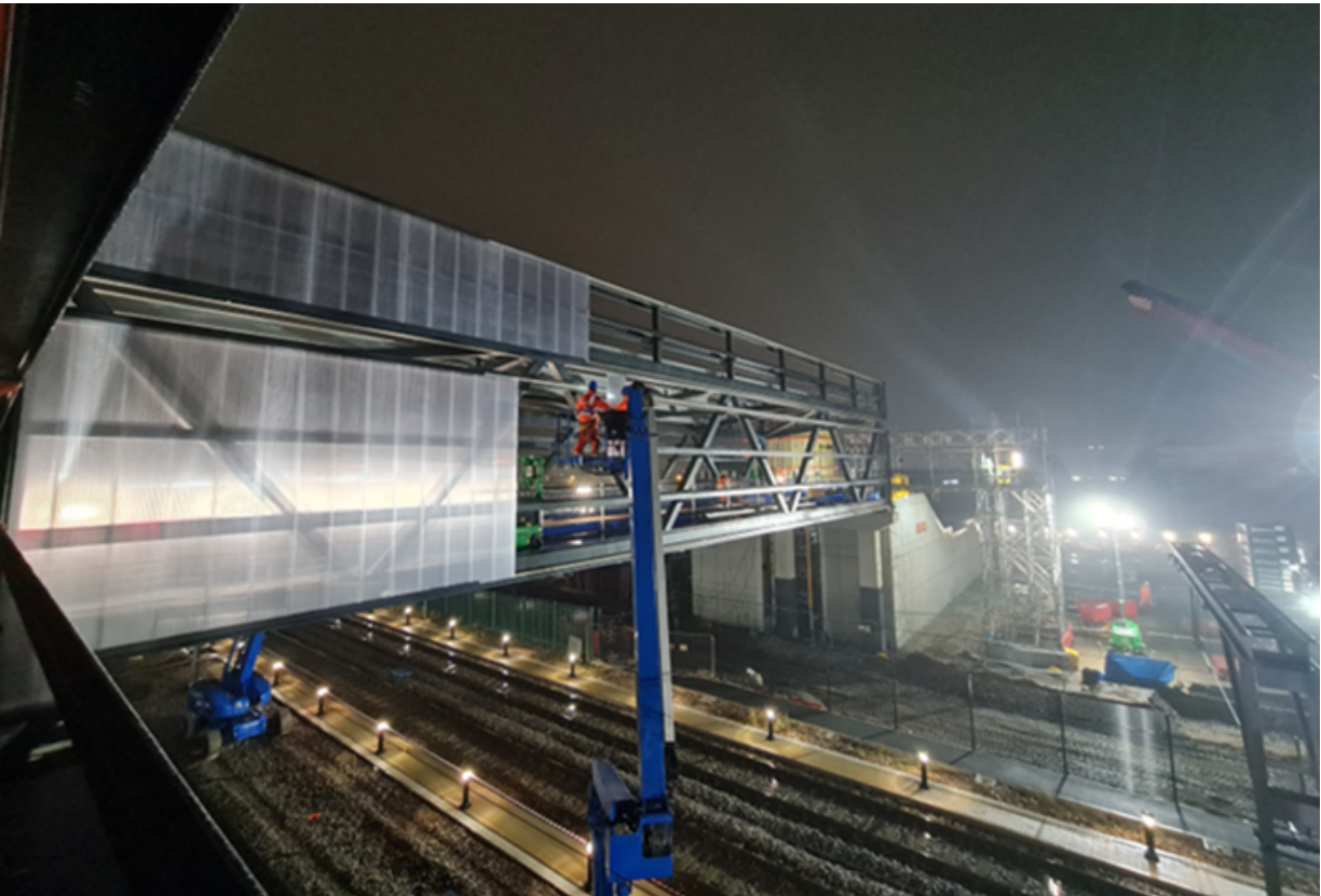
Footbridge cladding underway
