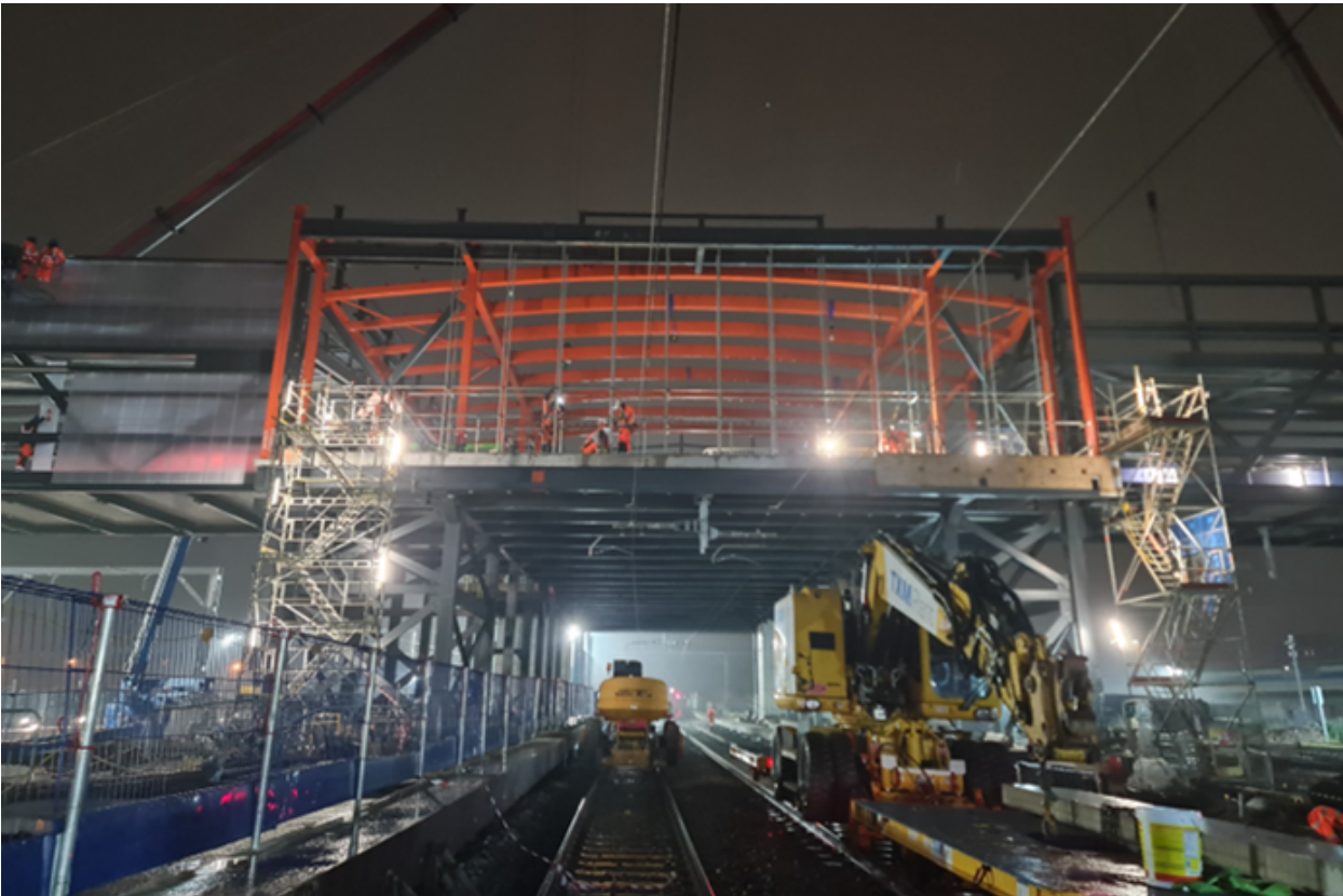
View of station concourse from below
